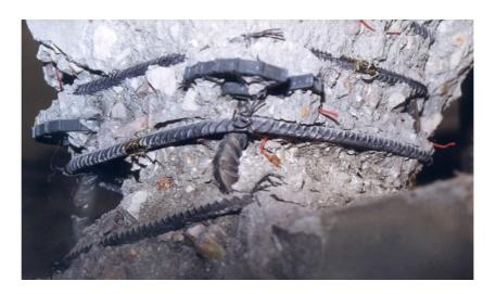
Typical failure of a column's upper part.
