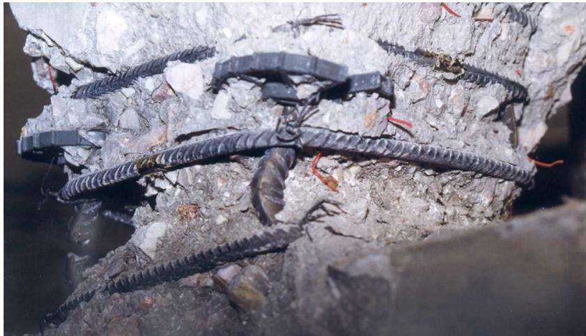
*Typical failure of a column's upper part.*
